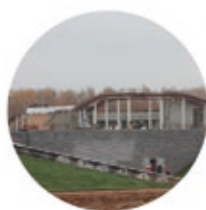
Power supply to the Skolkovo Innovations Center
